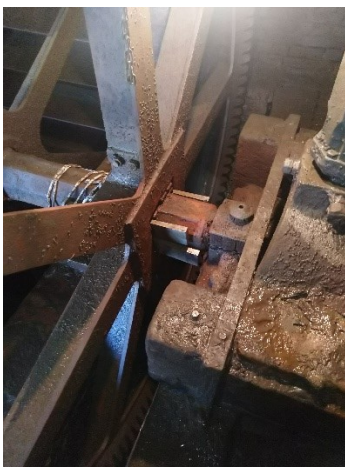
Figure 1 Work Under way
