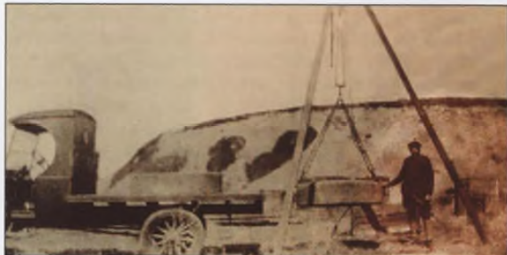
Fig. 15. Charles W. Snow removing the millstones (photograph from Snow family history in Highland House, Truro Historical Society, Truro, MA).
