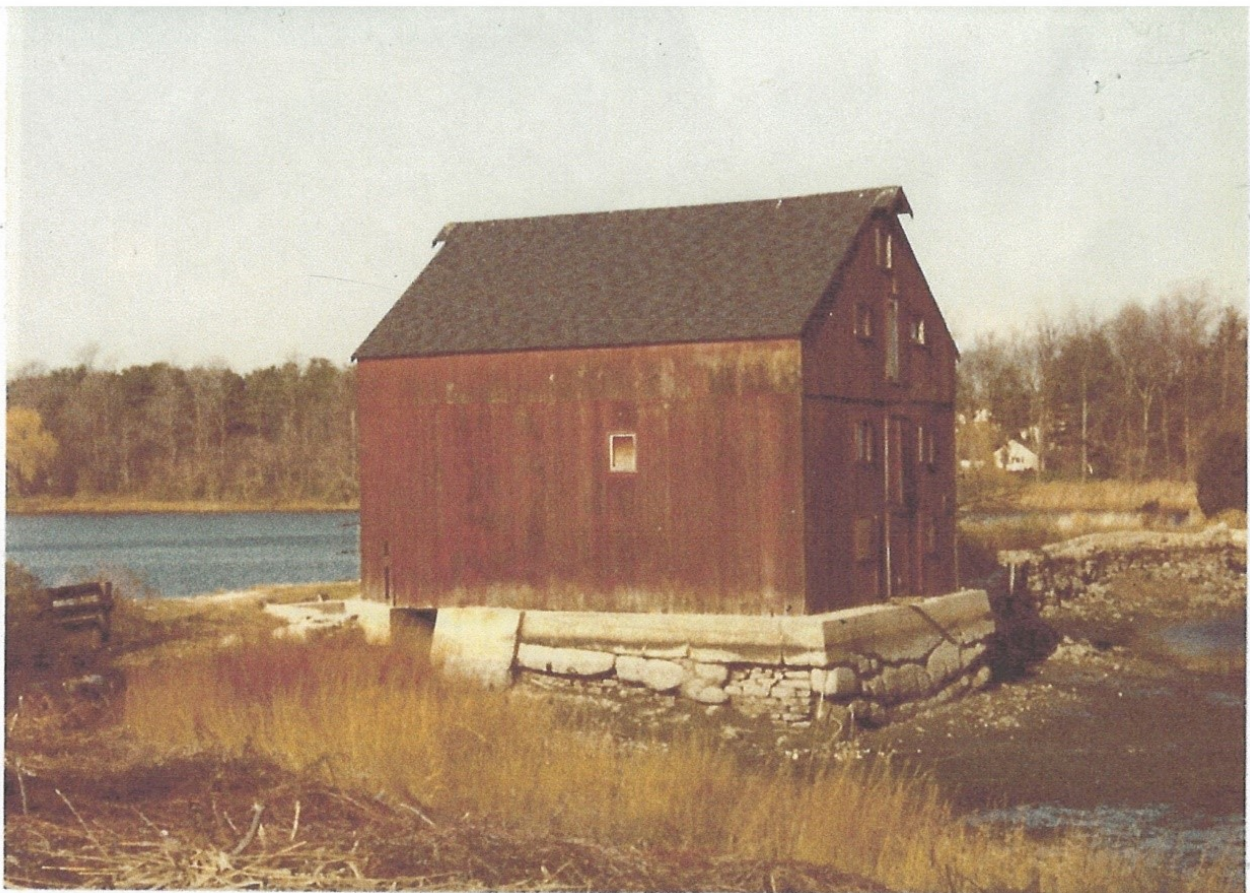
Deteriorated concrete encasement - 1983
