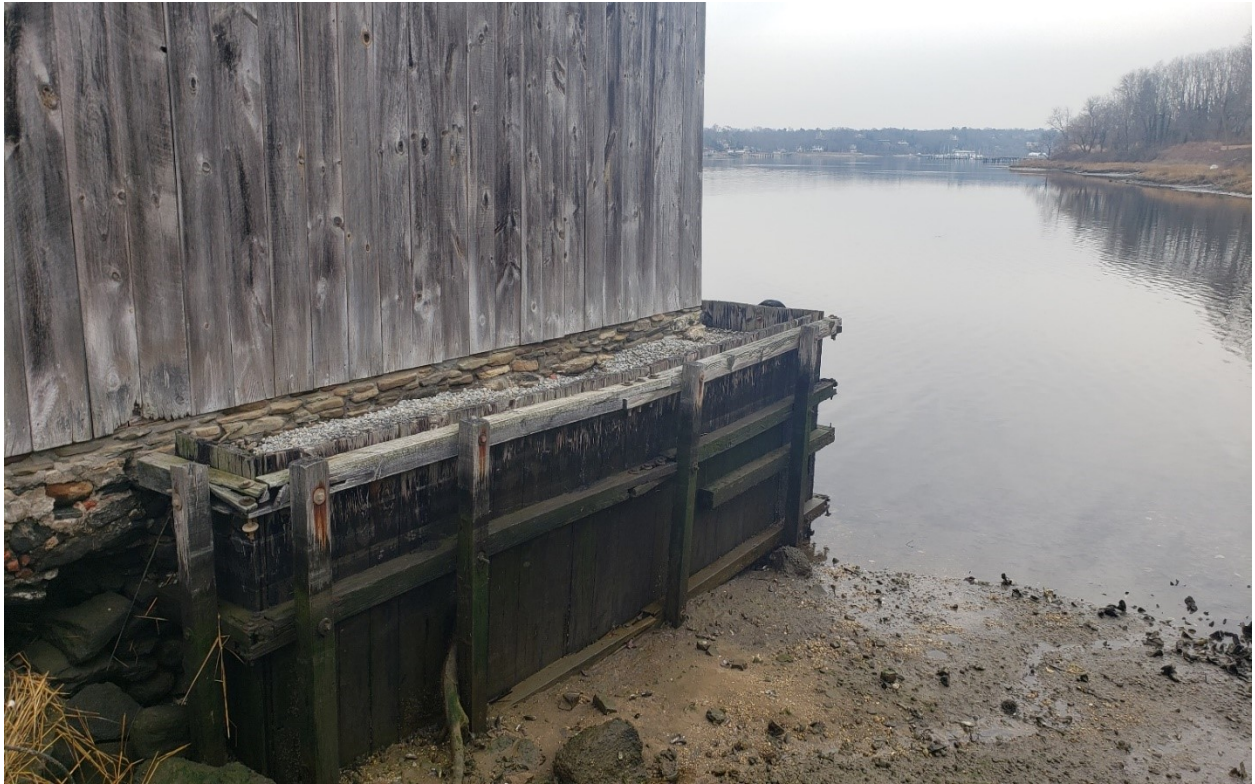
South facing bulkhead – 2020
